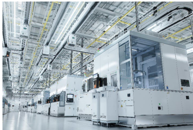
Factory / Plant Equipment
