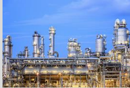
Oil Refinery, Petrochemical
