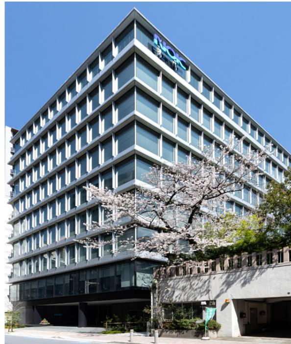
Glass is used on three sides of the building to efficiently utilize natural light
