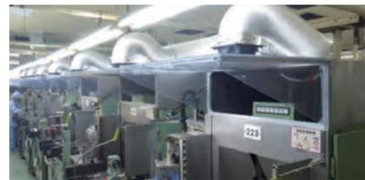
Figure 2: Individual heat exhaust hood
